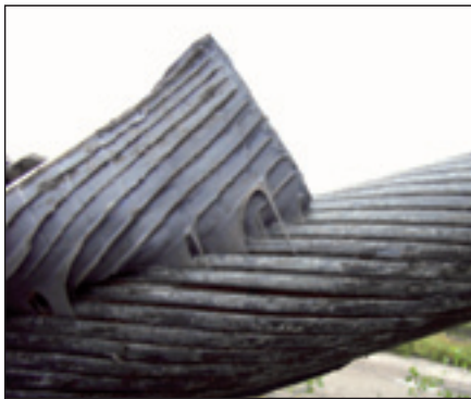
Adhesion of the tape on cable surface
