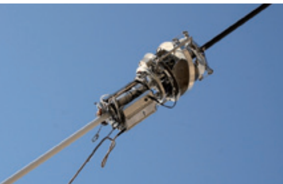
Automatic application of the corrosion protection system
