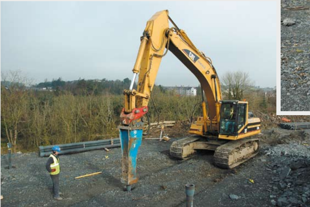
i Client PJ Edwards DSI Services Supply of 36 DYWIDAG Ductile Iron Piles, each 12-15 m long, non-grouted, technical support and site supervision
