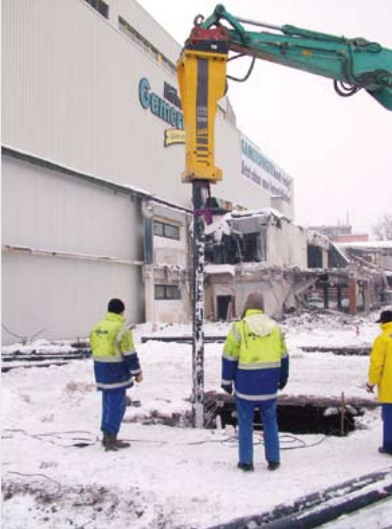
i Client Keller Grundbau DSI Services Supply of 332 DYWIDAG Ductile Iron Piles, 3.500 m, not-grouted
